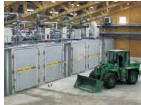
Intensive composting in Herhof composting boxes
