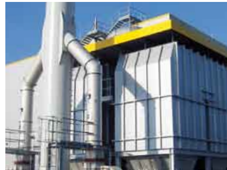
Construction of biofilters and thermal air purification plants (LARA®)
