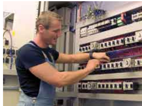
Construction of controlling and switching systems
