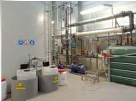
Construction of water treatment plants
